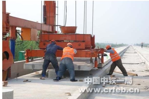
After the pretension process, cement is used to cover all the pretensioned steel bars. Once the cement is cured, the whole block of foundation will be cut into pieces which will then be installed on the railway line.
