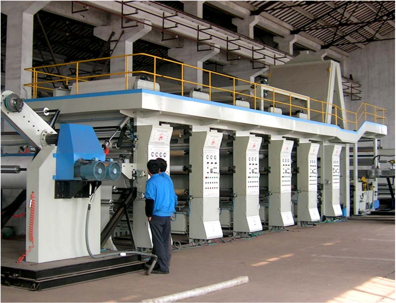
Five colour Printing press during commissioning.
